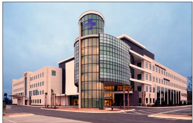
Figure 8. The 95,430 square foot Cancer Center of Sacred Heart Hospital in Pensacola, FL, completed in April 2010 as an addition to the original medical office building. The center was designed to meet Florida's coastal building code standards for hurricane and wind resistance utilizing the impact resistant version of Kawneer's 1600 Wall System®1 and IR 501 storefront framing system, with insulating laminated 15/16-inch impact resistant glazing (photo courtesy of Kawneer Company).
