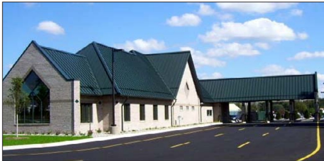
Figure 6. Metal roof on the Team One Credit Union building covering 11,500 square feet and built with Petersen Aluminum's 24 gauge 3105-H14 SNAP-CLAD panels pre-painted in Hartford Green (photo courtesy of Petersen Aluminum).
