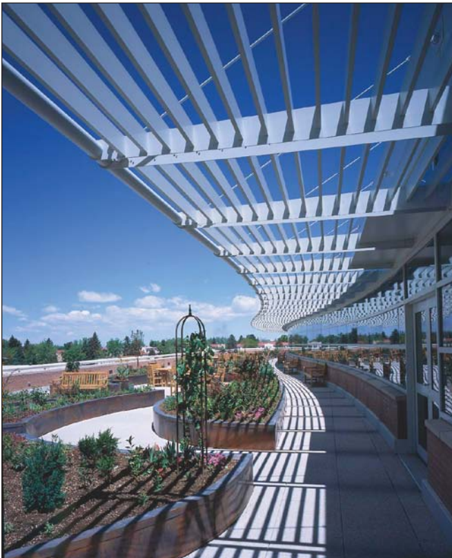
Figure 10. Example of Aiolite sun controls to shade windows at the University of Colorado Hospital in Aurora, CO.
