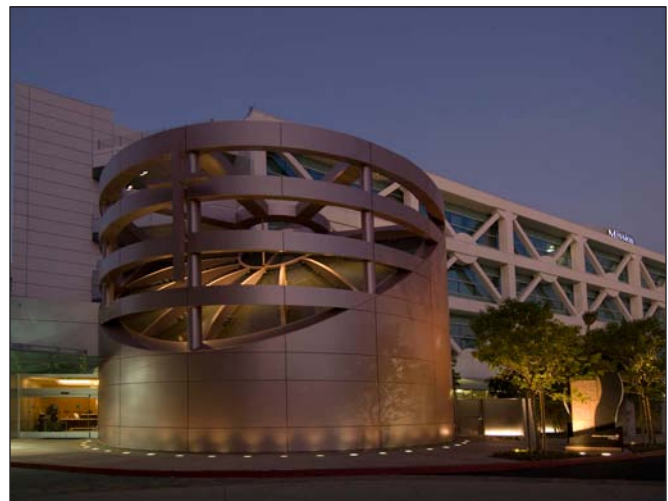
Figure 5. The Mission Hospital Chapel is clad in 4 mm thick panels of Alucobond aluminum composite material produced in the 3A Composites' Benton, KY, plant (photo courtesy of 3A Composites).
